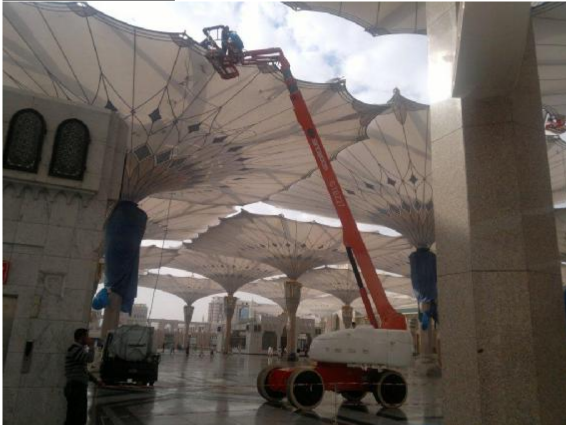
GTBZ20&25&38J&42J Working for stadium maintenance
